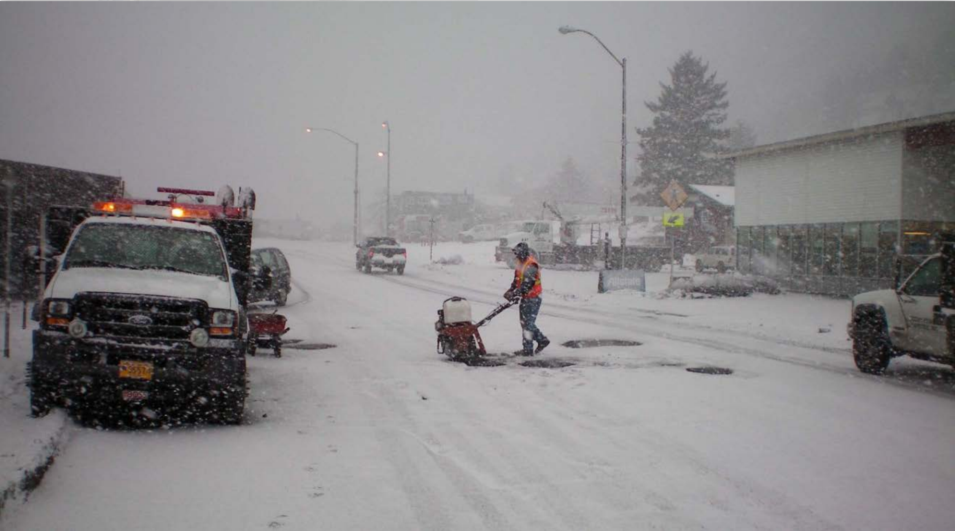
Filling potholes in the snow! Photo by Noah Hill, Alaska DOT&PF
