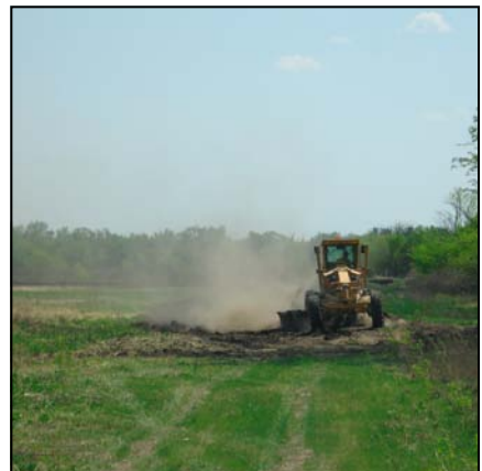
Road construction at Flint Hills NWR.
