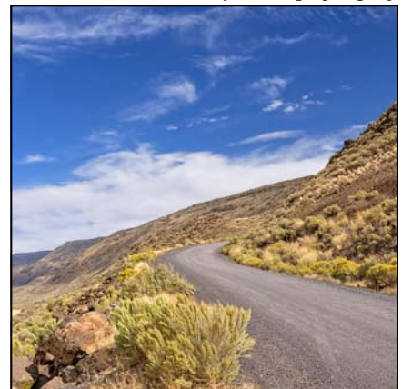
Roadway terraced along hillside at Hart Mountain NWR responds to opportunities and constraints of the topography
