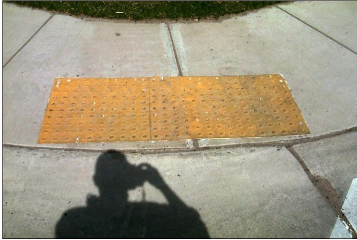
Installation 7: Located on the northwest corner of the intersection of 3 rd Ave. N. W. and 6 th St. N. W.
