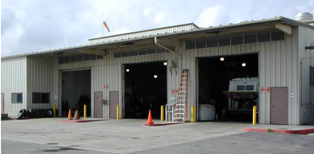
Figure C-10. CNG maintenance facility in Thousand Palms
